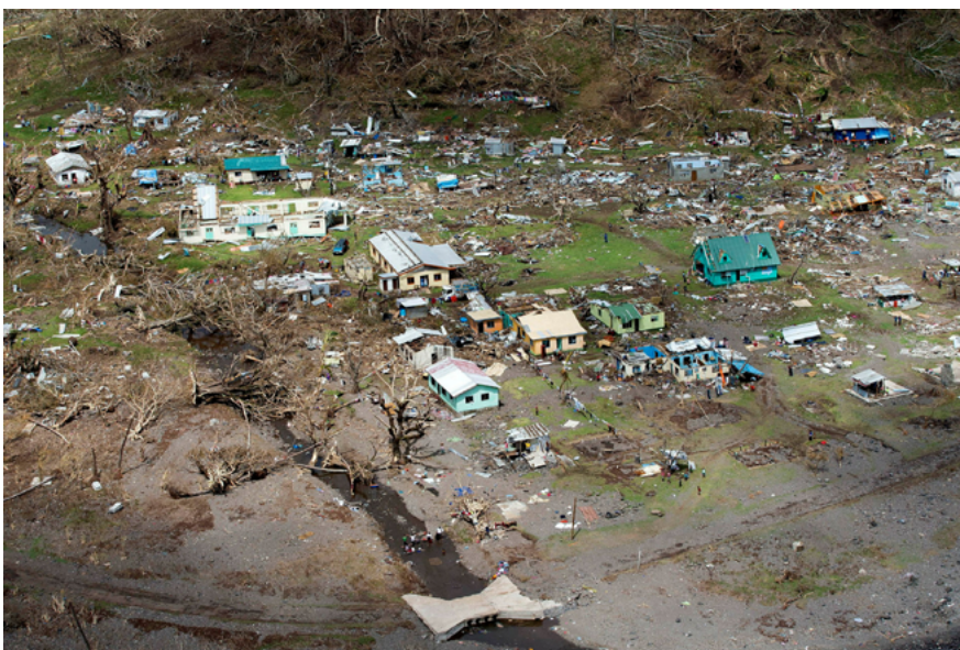
Figure 6. An aerial view of damage on Koro Island after Tropical Cyclone Winston (Source: Department of Defence) 180
