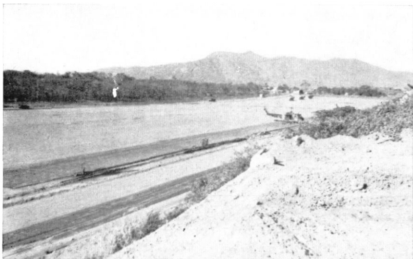
Kangaroo Helipad: 1 ATF Base. Reconstructed and sealed by 17 Construction Squadron RAE.
