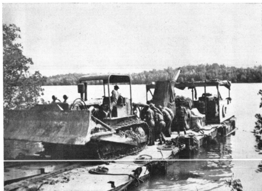
Unloading from the Unifloat at Simandalan Island.
