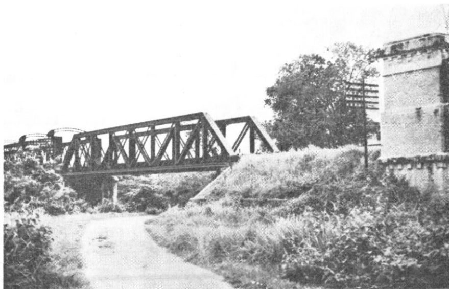
Victoria rail bridge, from west side. Original abutment at right and new span replaced by Japanese.
