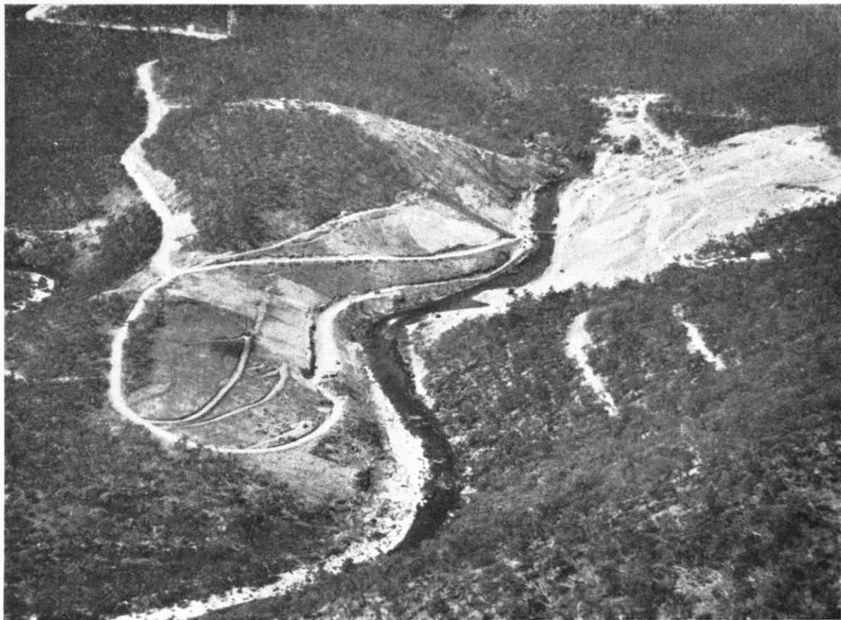
Aerial view of the site of the Adaminaby Dam.
