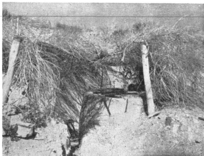
Concrete MG post hidden under thick camouflage of reeds.
