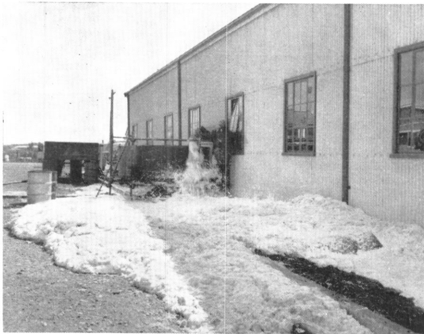
"Snow" from the foam pump test in the Mechanical Test House at Maribyrnong.
